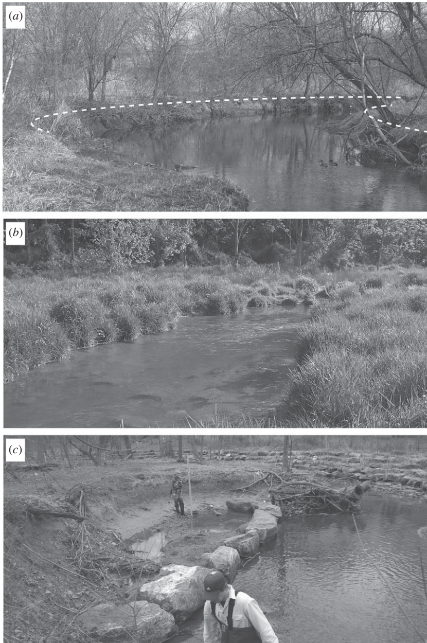
Figure 11. (a) Lititz Run before restoration, in 2001, with high banks of millpond sediment exposed along the incised stream upstream of a breached milldam (photograph by Ward Oberholzer). (b) Lititz Run in 2007, after approximately 23\,000\text{ m}^3 of historic sediment was removed to a depth of about 0.5 m above the pre-settlement valley bottom along the stream corridor. Note wetland sedges and other plants that grew in the exhumed wetland conditions soon after restoration. (c) Conventional approaches to stream restoration generally consist of attempts to stabilize meander bends with hard structures, even on incised streams near breached milldams in small headwater areas of streams, as here at Woottens Mill park restoration (completed 2006) along Watts Branch, MD. (Photograph taken March 2008.)
